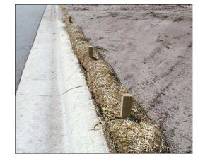
Wattles (also called bio-rolls or sediment logs) are made of straw or wood fiber bound within a net to form a tube. They typically come in 10 foot lengths and are 9-20 inches in diameter.
